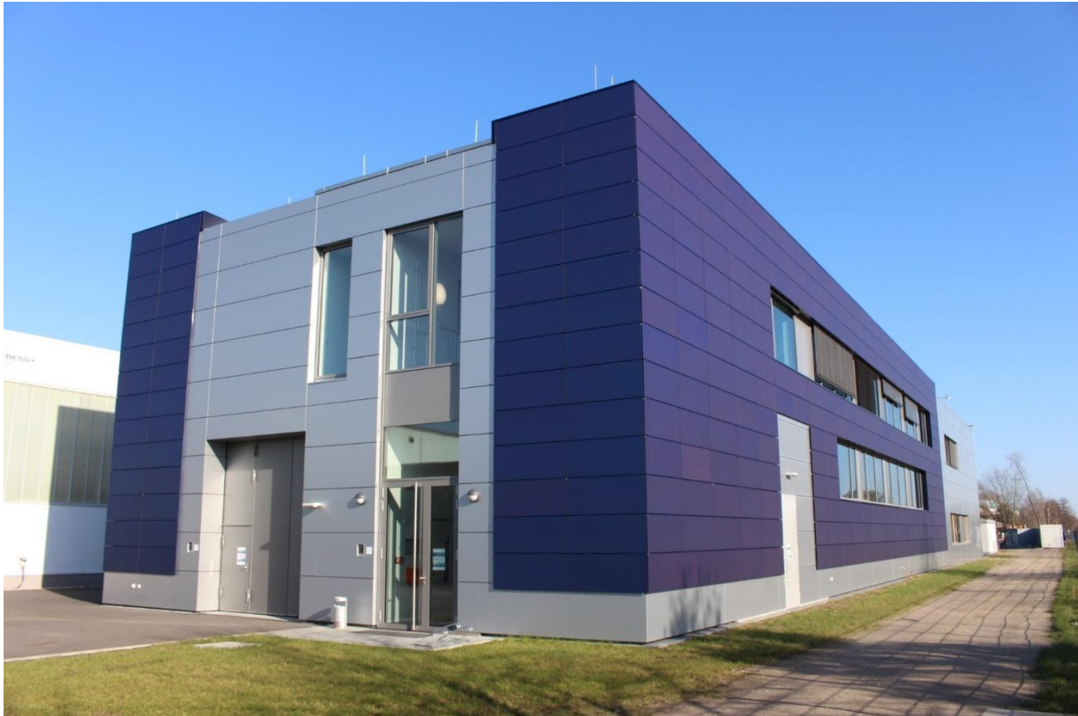
Figure 2: HZB Living Lab for Building-integrated Photovoltaics (South-West view)
