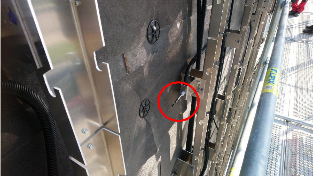
Figure 8: Placement of the air flow measurement device during the construction process
